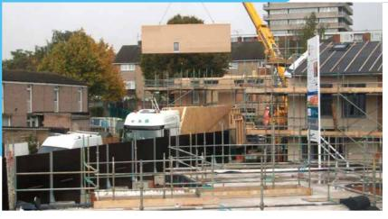
Sampson Close, Coventry. Main frame, insulation, doors and windows constructed as panels off site. Architect: Baily Garner.
