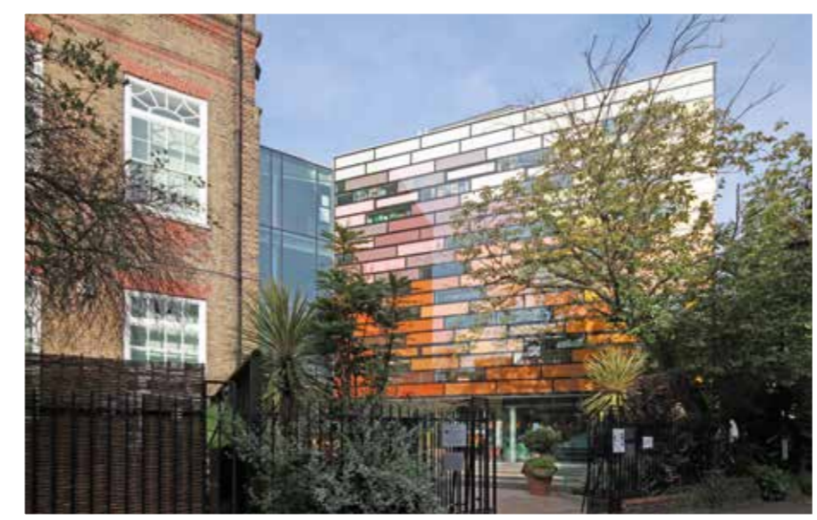
Clapham Manor Primary School. Managing repairs to curtain walling.
