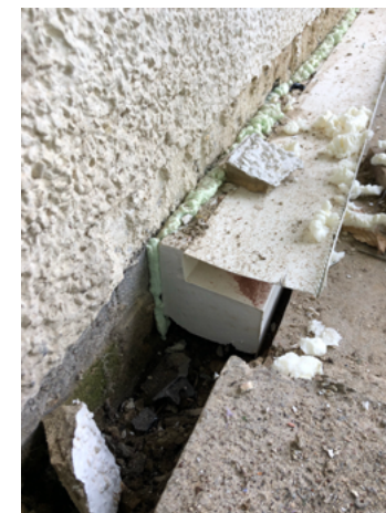
Figure 17 - EWI starter track
