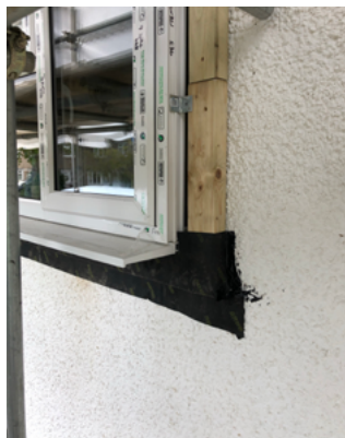
Figure 24 - Airtightness tape
