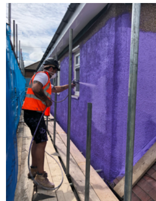
Figure 26 - Spray applied liquid membrane
