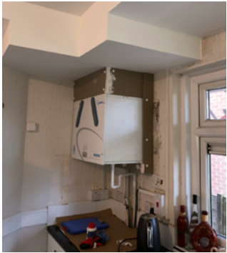
Figure 36 – Mechanical Ventilation with Heat Recovery (MVHR)
