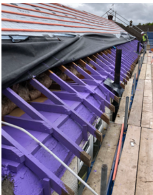
Figure 23 - Brush applied liquid membrane
