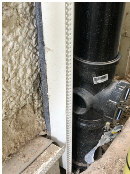
Figure 30 - use of aerogel insulated track to avoid reducing external access
