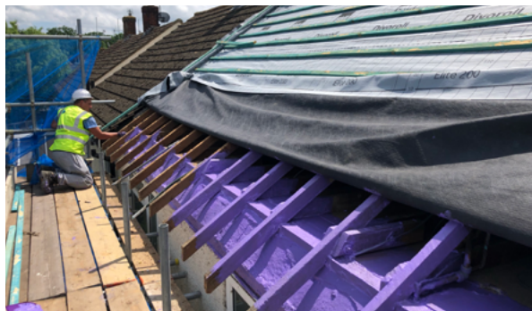
Figure 22 - Brush applied liquid membrane
