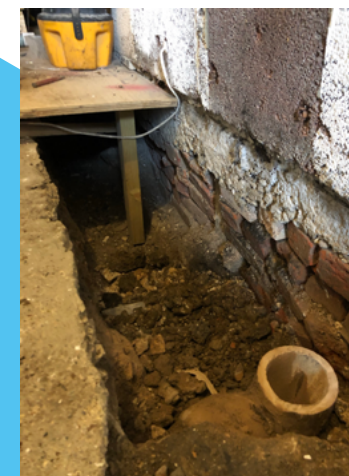
Figure 18 - Excavation for EWI
