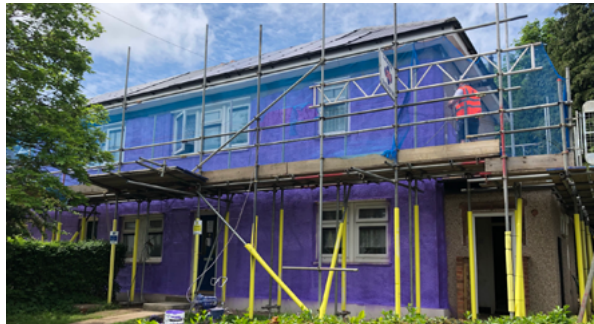
Figure 21 - Spray applied liquid membrane
