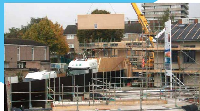
**Sampson Close, Coventry.** Main frame, insulation, doors and windows constructed as panels off site. **Architect:** Baily Garner.
